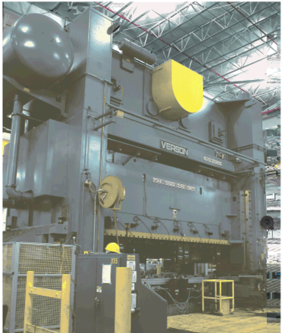
Isolators installed, press leveled, and aligned in five hours!
